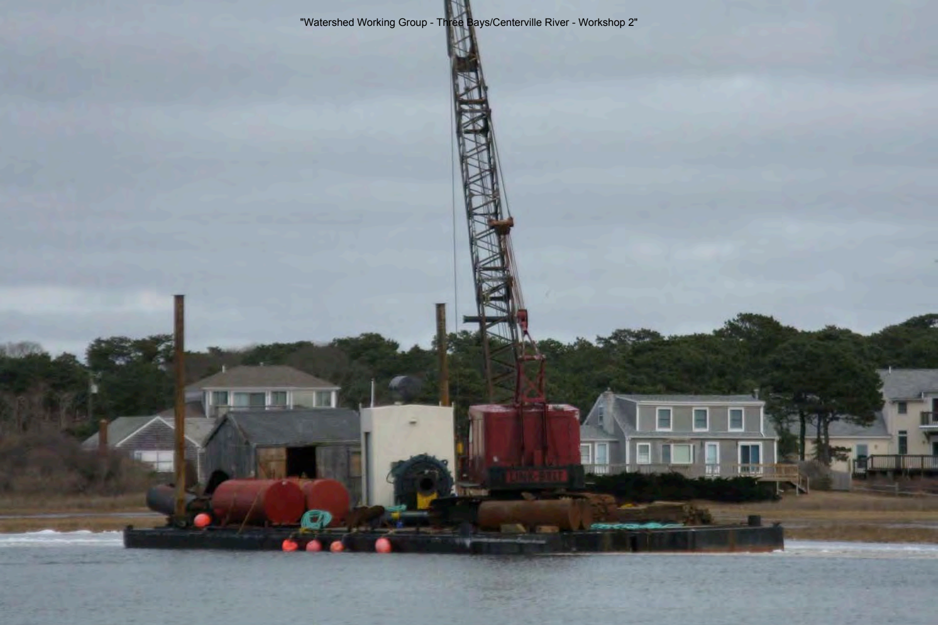
Precedent: Pond and Estuary Dredging - Dennis, MA Source: Cape Cod Times
